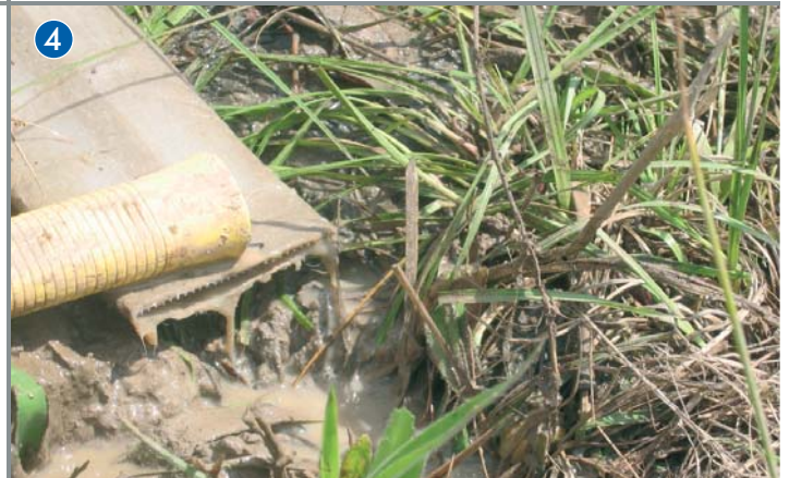
Drive Plati-Drain® into optimum position
