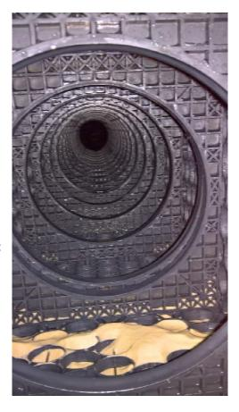
Maintenance Ports / Inspection Ports: Maintenance/inspection ports are located near the inlet and outlet connections, treatment rows, and throughout the system. These should be used to check for sediment and typically allow access for backflushing and cleaning.
