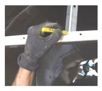
7) Mark the center of the bracket on the back (pipe side) edge.
