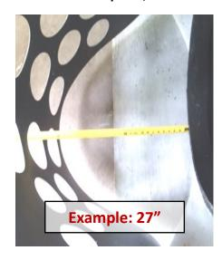
12) Subtract the greater of 15" or half the pipe diameter from the measurement in Step 11. Mark that distance on the dissipator from the wall and draw a vertical cut line. Cut line must be at least 1.5" from any Dissipator opening — adjust as necessary.
