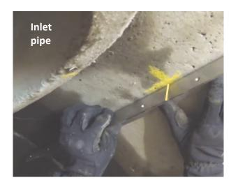
8) Align wall bracket with marks made in Steps 5, 6 and 7. Use level to ensure bracket is vertical prior to next step.
