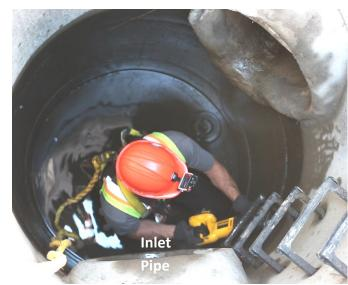
5) Make a vertical mark 9" ± from inside of pipe. Repeat on other side of pipe at an equal distance.
