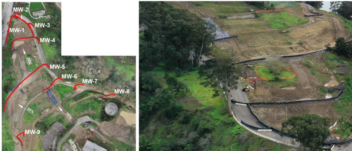
Figure 3. Aerial view (left) and side view (right) of the barrier wall basin locations.
