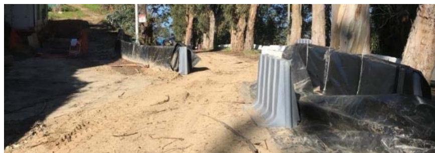
Figure 11: Empty barrier walls set aside for haul road use.
