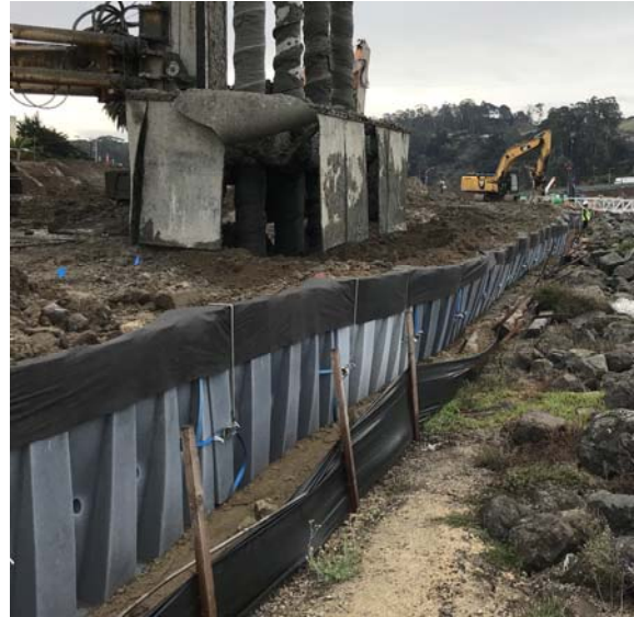
Muscle Wall as a temporary retaining wall for soil
