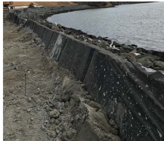
Muscle Wall as a liquid waste containment barrier
