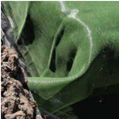
Figure 17: fold corners flat against the tank
