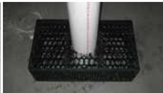
Figure 13: Place inspection port into underdrain module
