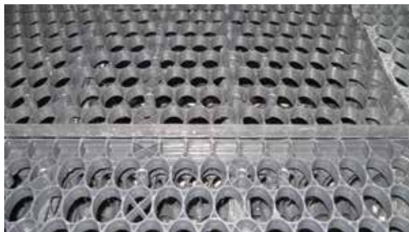
Figure 9A: Minor Variations (less than width of top plate) in tank height are acceptable
