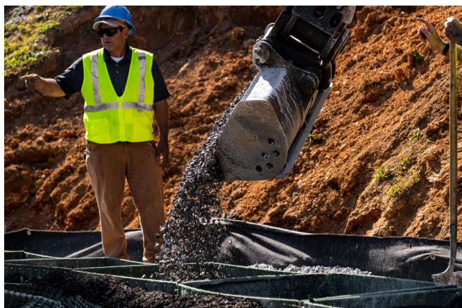
Figure 3: Coarse gravel infill used in base row of PROPEX Scourlok
